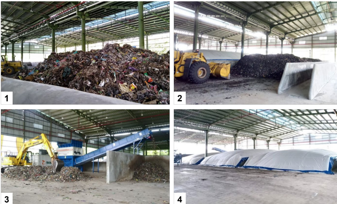
Figure 30: MSW to RDF pre-processing facility in Tritih Lor Village in Java [76]
