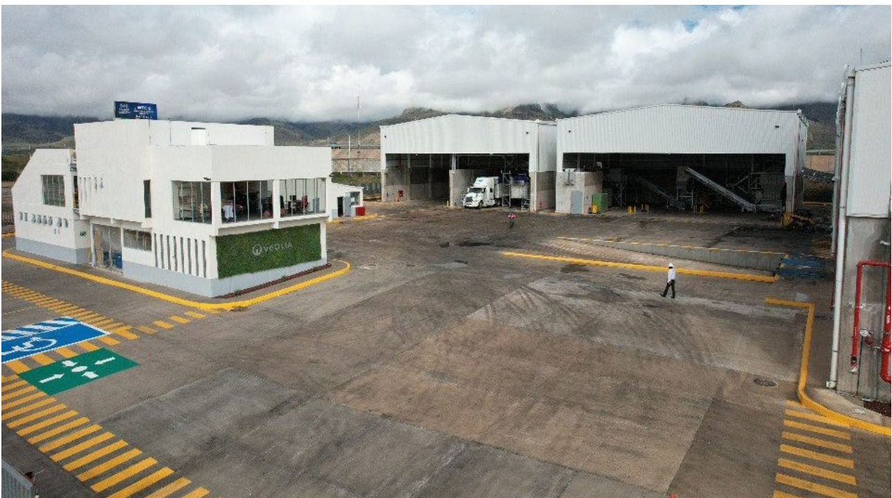
Figure 34: RDF pre-processing plant, exterior view, San Luis Potosí, Mexico [78]
