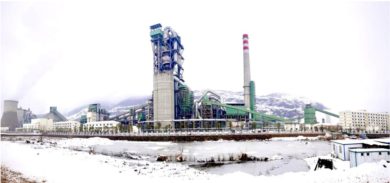
Figure 29: RDF co-processing cement kiln system, Huangshi city, Hubei province [75]
